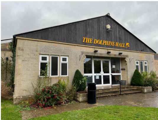
Dolphins Hall Front entrance
